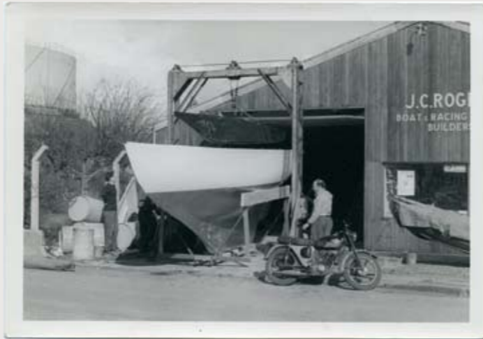
Left Jo Mooring-Aldridge's Sulali dries out, showing the Contessa's deep and long keel with its horizontal base, which many believe is a marked improvement on the Folkboat. Top Jeremy Rogers built his first Folkboat in a garage beside his house in Lymington. Extracting it was tricky. Above The first Contessa 26 hull emerges from Rogers' first Lymington factory.
